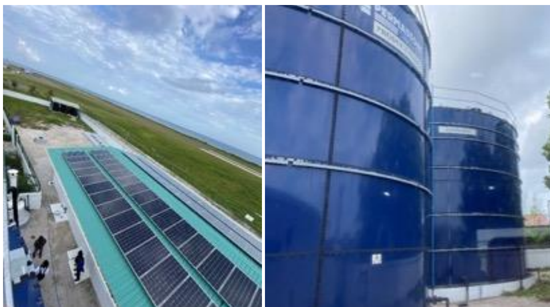
Figure 1. Combined rainwater and reverse osmosis water plant serving island communities
